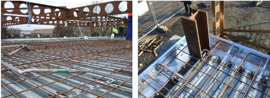
Fig. 3.6. Mesh reinforcement and steel decking before concrete casting (MACS+, RFCS, 2014)
