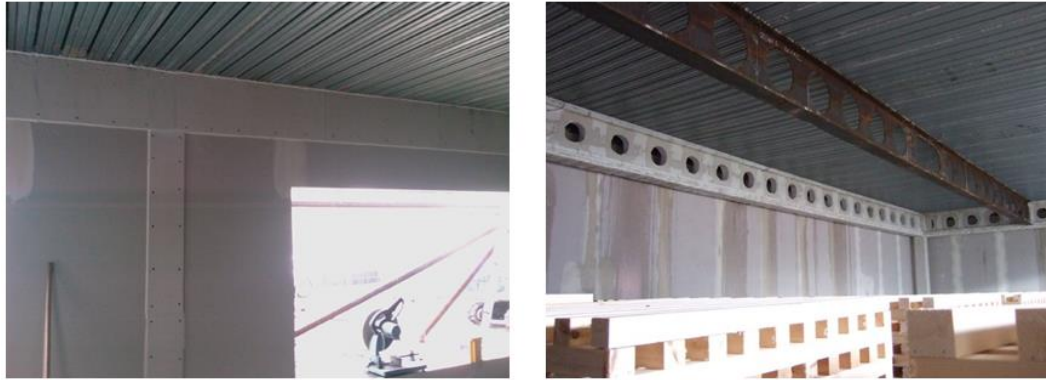
Fig. 3.5. Fibre and plasterboard protection used inside the compartment (MACS+, RFCS, 2014)
