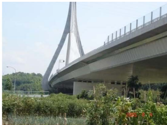
Figure 5. Pedestrian bridge with curved SIN-beam and the span of 42 meters and width 2.25m, Almaty, Kazakhstan
