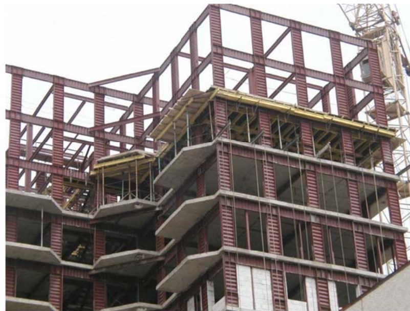
Figure 4. Application for the first 15 floor residential building with the seismicity of 9, Kazakhstan 2005 (The Medvedev–Sponheuer–Karnik scale)
