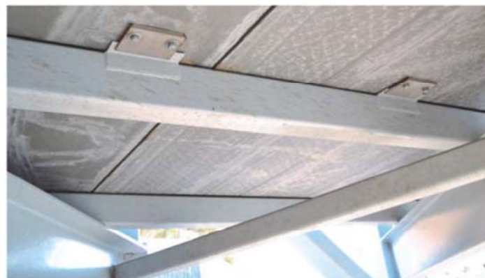
Figure 29. Connection of the fiberglass panel to the structure.
