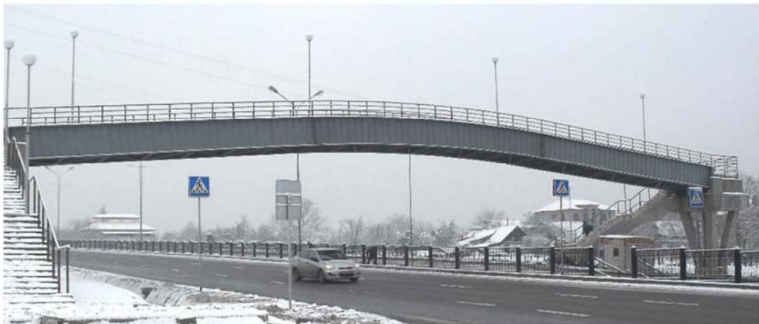
Figure 5. Pedestrian bridge with curved SIN-beam and the span of 42 meters and width 2.25m, Almaty, Kazakhstan
