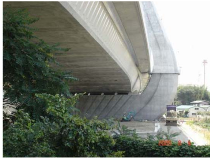
Figure 6. Yahagigawa composite cable-stayed bridge with the span of 235 meters, Japan
