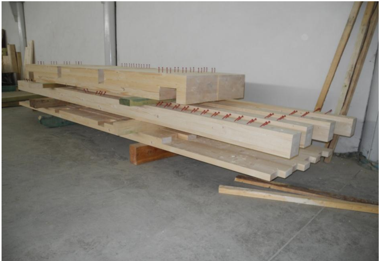
Assembled timber frame of the slab with formwork
