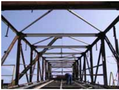
Replacing of the end frame
