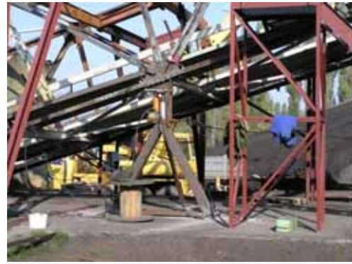
Straightening of frame geometry
