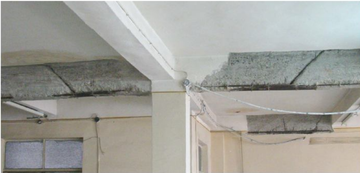
The clean surface ready to strengthening
