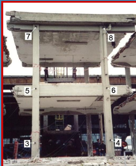
Displacement measuring devices
