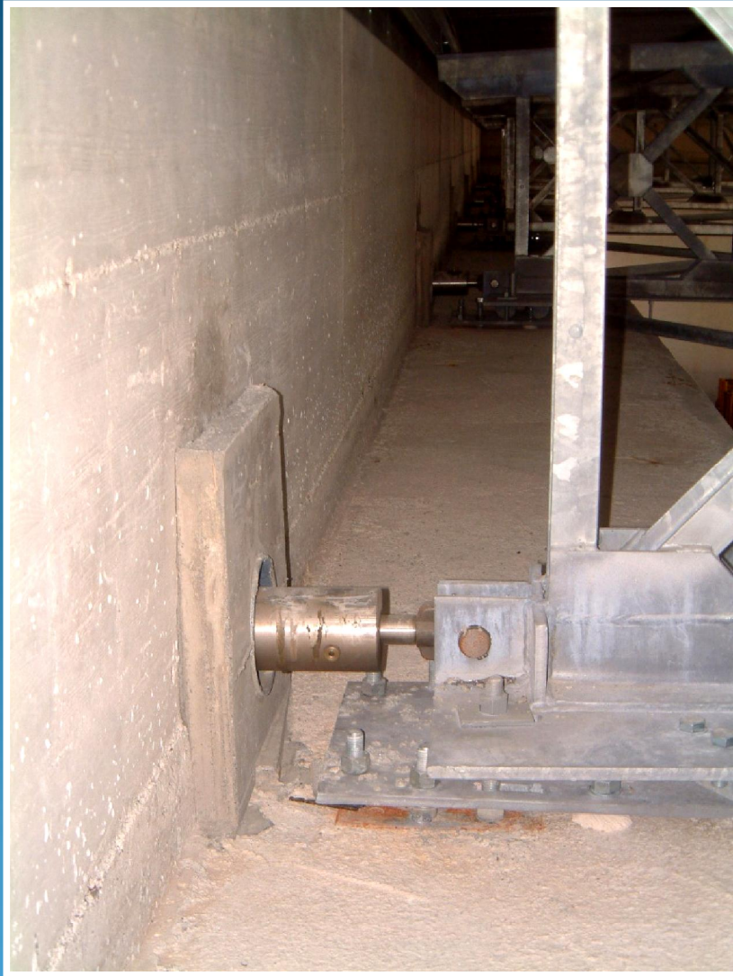
North side device : 12 shock transmitters
