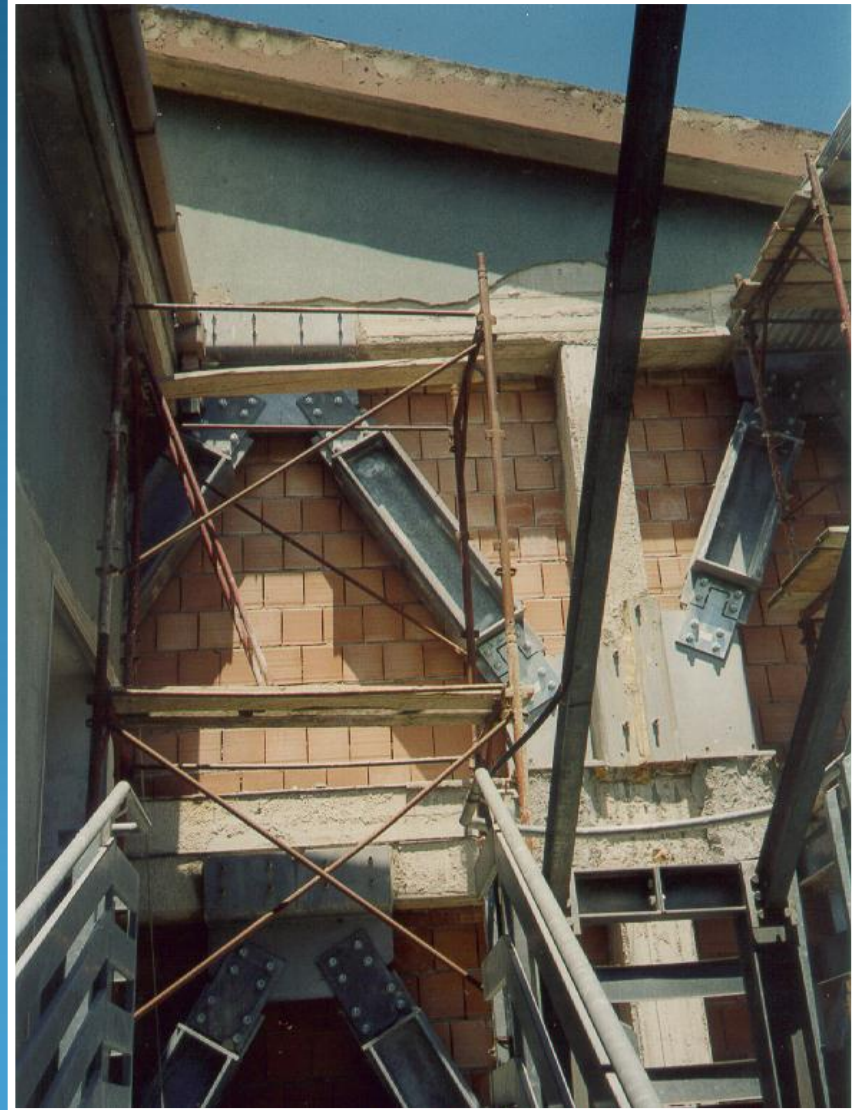
Dissipative braces in two schools in Potenza
