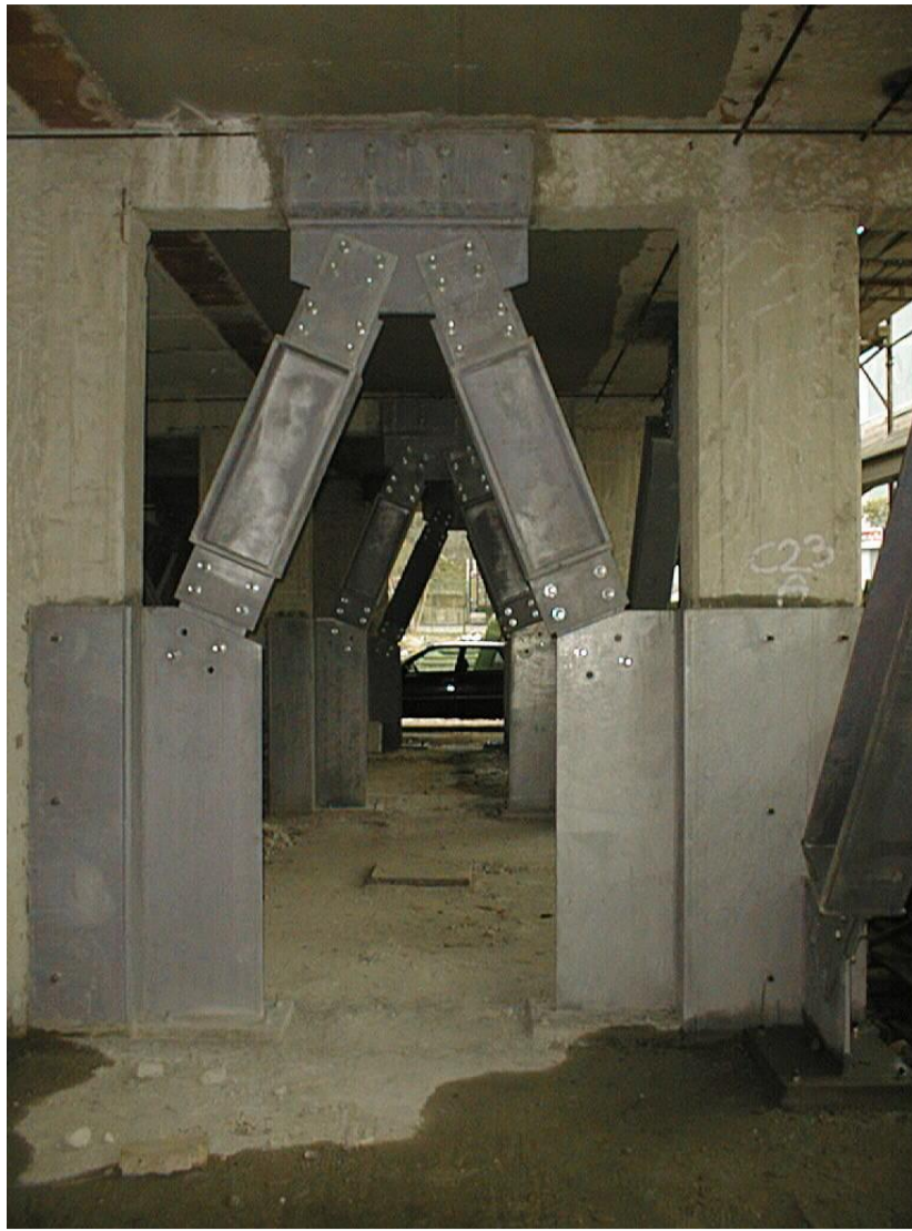
Dissipative braces in two schools in Potenza
