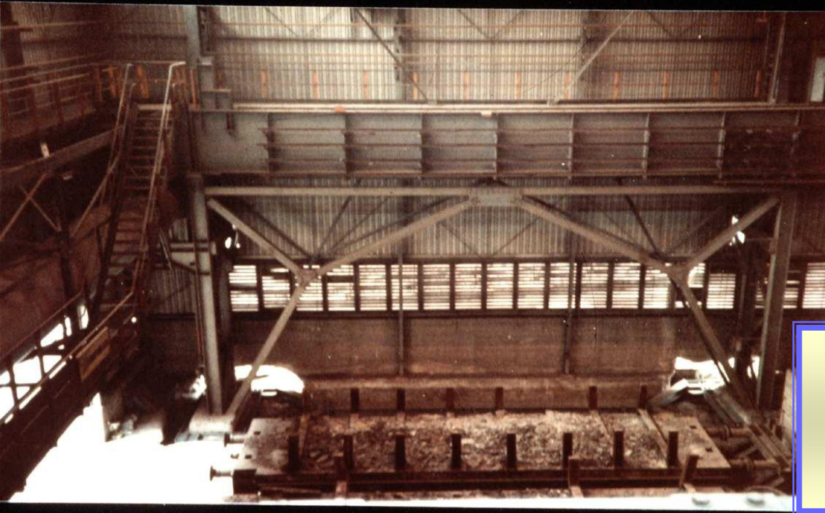
ILVA steel mill (Bagnoli - Naples, Italy): seismic upgrading
