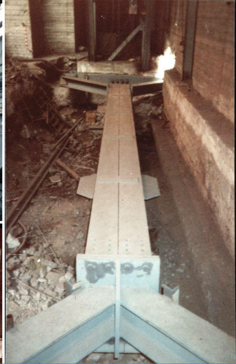
ILVA steel mill (Bagnoli - Naples, Italy): seismic upgrading
