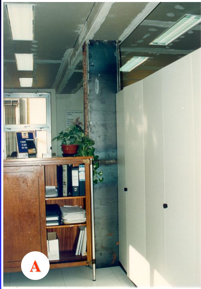
reinforcement with steel plates and in-filled concrete
