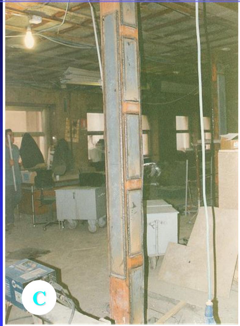
steel plates, in-filled concrete and Dywidag bars
