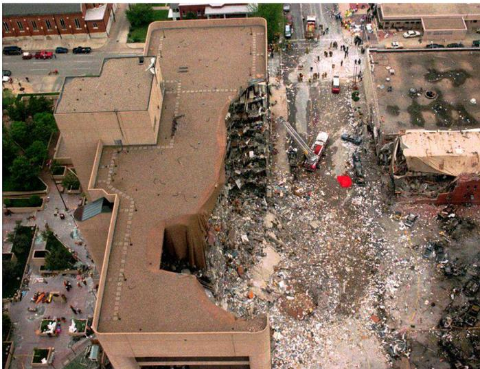
Figure 2 Murrah building collapse
