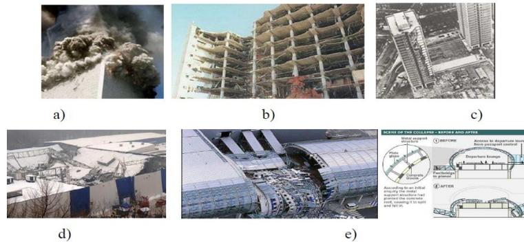
Figure 1.6 Progressive collapse: a) aircraft impact at WTC, 2001; b) Oklahoma City bombing, 1995; c) gas explosion at Ronan Point building, 1968; d) snow accumulation at Katowice/Poland, 2006; e) wrong steel-concrete connection details at Charles-de-Gaulle Airport new terminal, 2004
