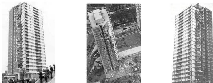
Figure 1.9 Ronan Point building after the collapse in 16 May, 1968 ([www.911research.wtc7.net](http://www.911research.wtc7.net))
