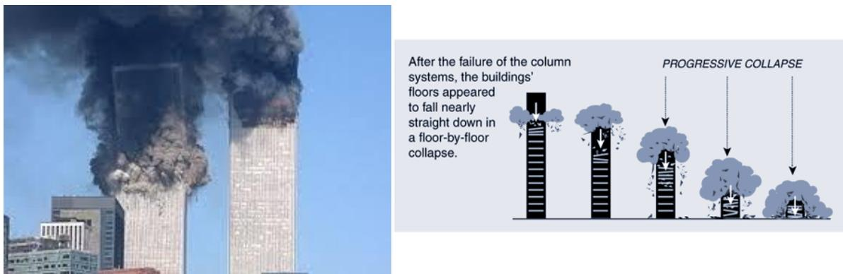
Figure 1.11 World Trade Center 1 and 2 collapse on 11 September, 2001 (www.wikipedia.org and www.911research.wtc7.net)
