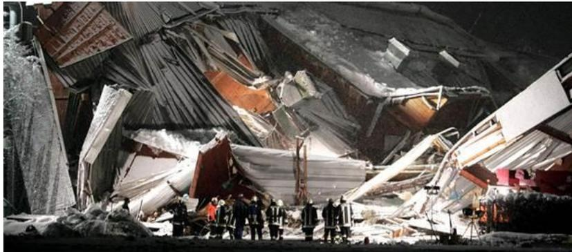
Figure 1.1 Failure of the Bad Reichenhall Ice Arena, Germany, 2 January, 2006 ([www.worldofkj.com](http://www.worldofkj.com))
