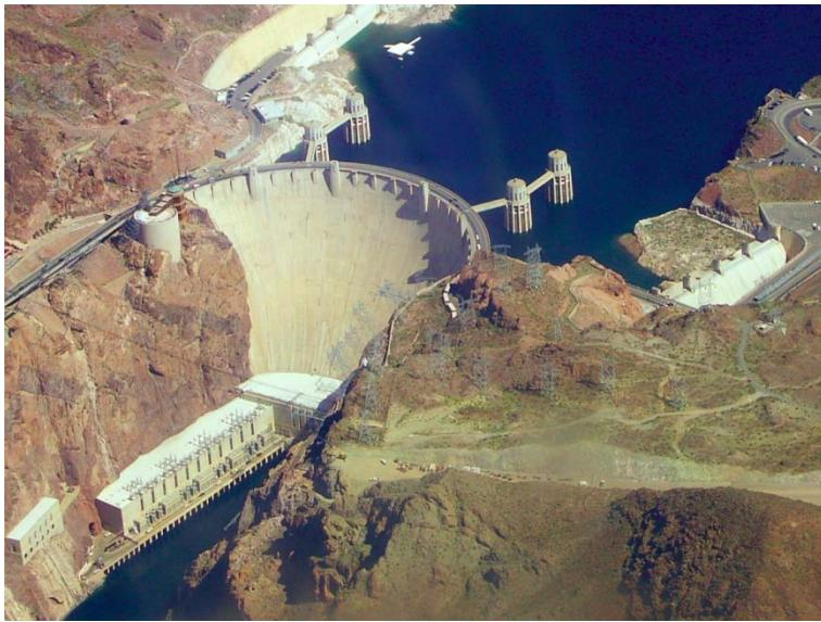
a concrete arch-gravity dam, built in 5 years
