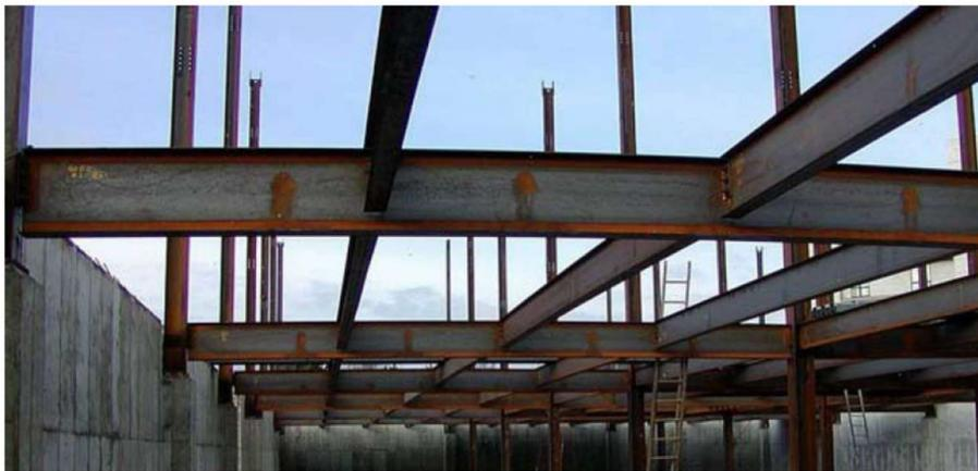
Figure 40. Serviceability condition of a floor system can be controlled through camber (curve of the beam in the vertical plane) at the time of construction
