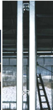
Pitched roof portal frame made by built-up sections (back-to-back C bolted connected by stitches,;
