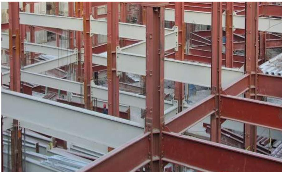
Figure 51. View of a steel frame structure, with cruciform columns and I shape beams
