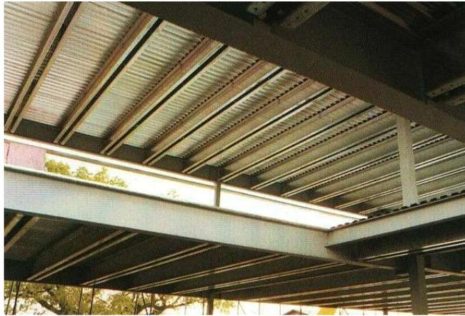
Floor structure: joist and sheeting on hot rolled steel framing structure
