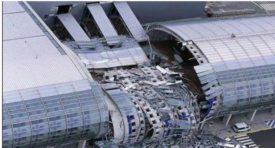
Wrong steel-concrete connection details at Charles-de-Gaulle Airport new terminal, 2004
