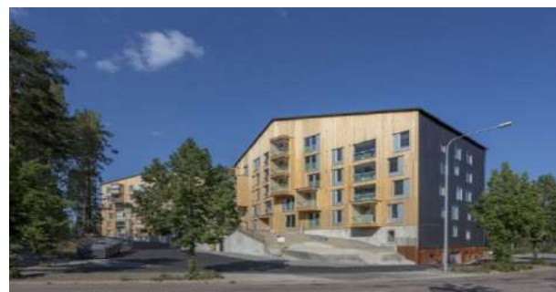
Figure 8. Puukuokka Housing Block (Finland) [5]
