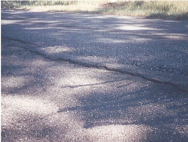
Fig. 2. Cracking with settlement
