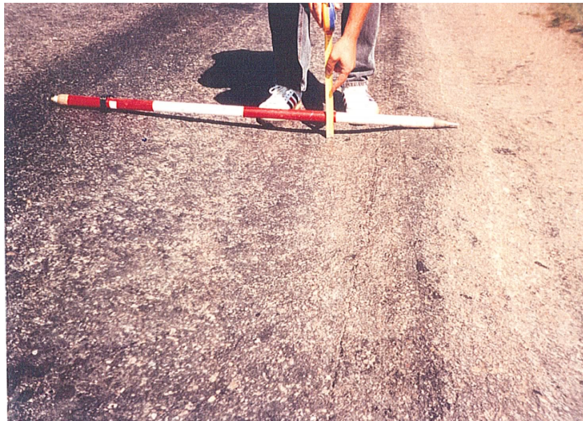
Fig. 2. Cracking with settlement
