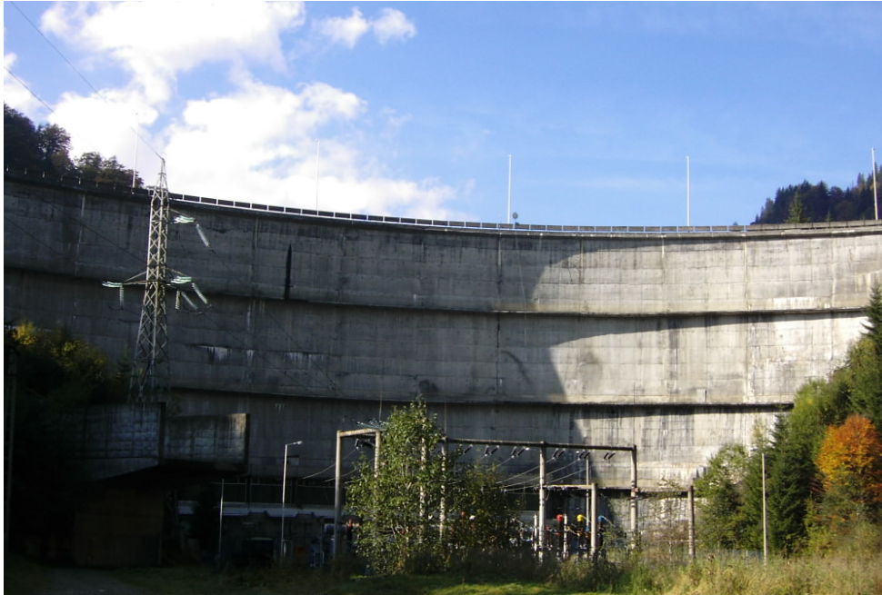
Fig. 2 Petrimanu dam overview
