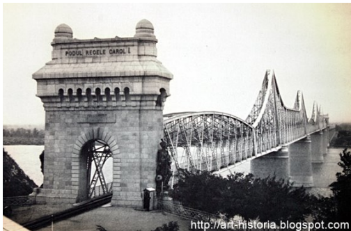
Fig. 1 Bridge King Carol I
