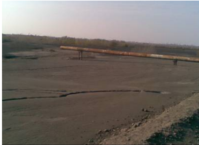
Fig. 1 The transportation of dense slurry into fly ash dump
