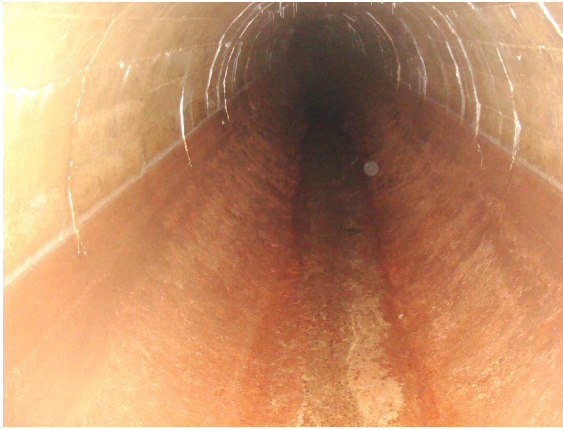
Fig. 2 View of the flow section of Strunga hydrotechnical gallery.
