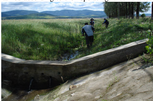
Photo 3 – Main drainage channel CP41 threshold drop of concrete, works for the destruction of aquatic vegetation and grassy (2010)
