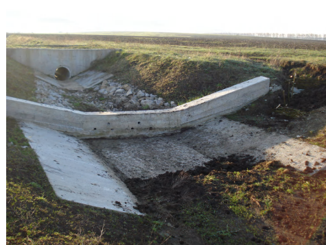
Photo 10 – Pipe culvert DN800 and threshold drop at drainage channel CS410 (2009)
