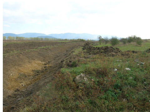
Photo 14 – Secondary drainage channel CT40321 (2008)
