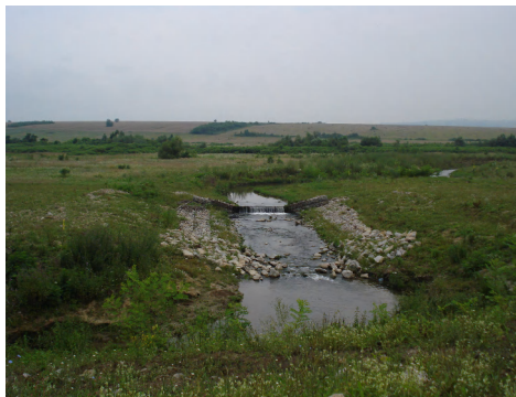
Photo 21 – Drop from gabions with rough stone on Lisava Valley at km 5+800 (2010)
