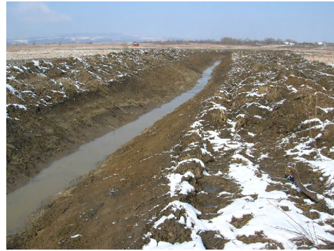
Photo 12 – Drainage channels CCS42 during execution (2008)
