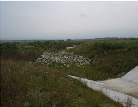
Photo 19 – Channel CP41 Consolidation with rough stone at the junction with channel CS410 (2010)
