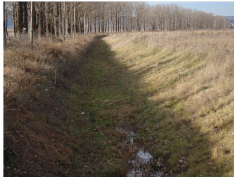
Photo 6 – Main drainage channel CP41 (2010)
