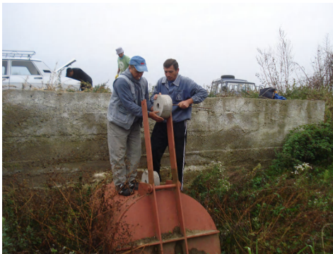
Photo 7 – Under-crossing the dike with metallic dampers Channel CCS42 Lisava Valley Maintenance and repairs works to the metallic damper counterweight (2010)
