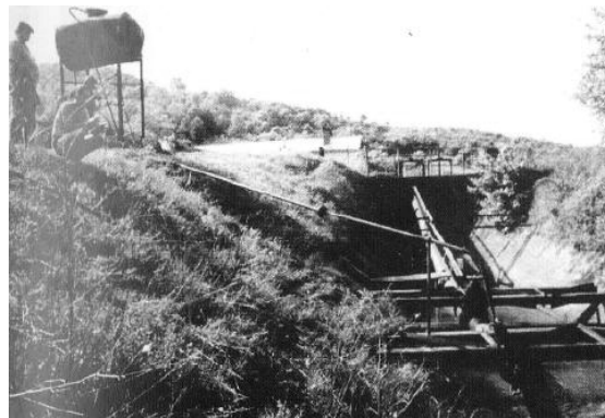
Fig.7 The pumping microstation Mocrea, Ineu, Arad county, Romania
