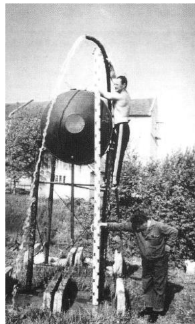
Fig.8 Storage tank at about 4m above irrigation ground level with a leveling staff
