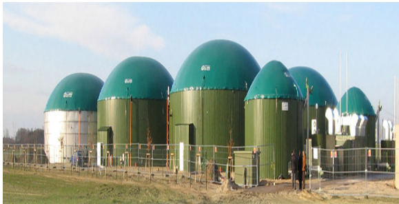
Photo 1. Digesters for anaerobic fermentation
