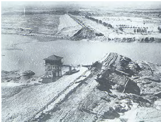
Fig.3 Banqiao Dam after the break.
