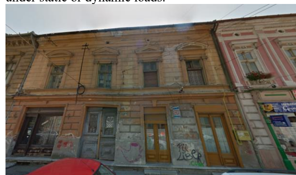
Figure 6. Pre-demolition state of the building
