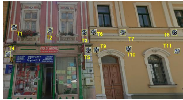
Figure 10. Placement of Topographic Targets
