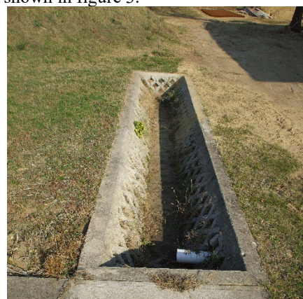
Figure 3 Gutter for rainwater infiltration into the soil, made of perforated tiles.
