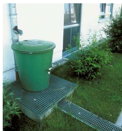
Figure 1.a Plastic tank placed above a gutter covered with a grate.
