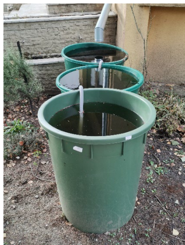
Figure 1.b Plastic tanks connected with siphon pipes.
