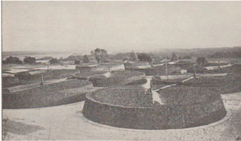
Figure 5. Trickling filters, treatment plant Wilmersdorf, ([1], p.p. 746)
