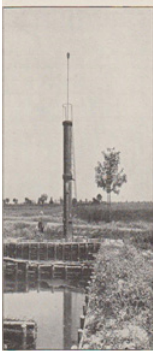
Figure 6. Settling ponds and infiltration fields, Berlin-Malchow area, ([1], p.p. 772)
