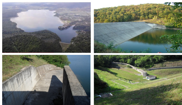
Figure 2. Surduc reservoir and dam
