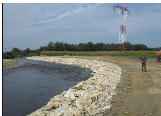
Figure 7. Consolidation of the right bank downstream of Curtea locality
