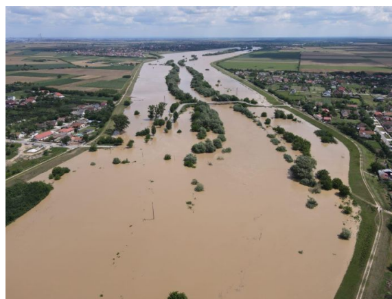
Figure 1. Breach in Dam , Timis River
