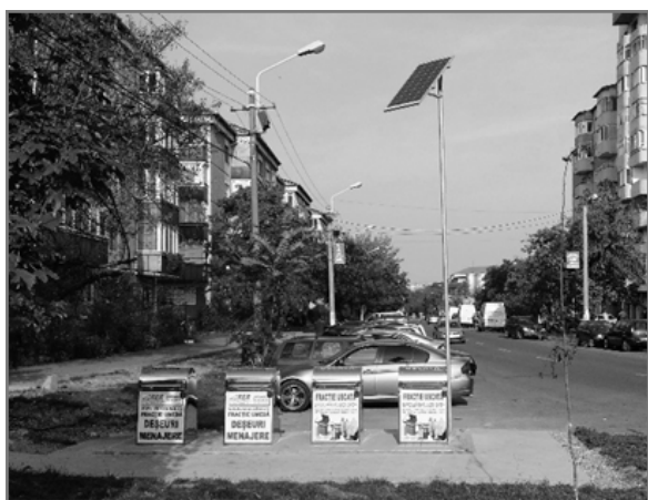
Figure 5. Underground platform with container monitoring and warning system
