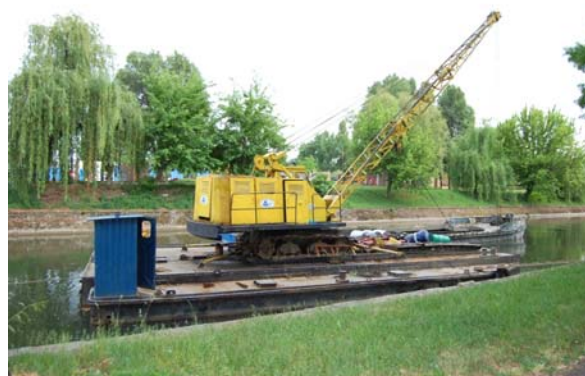
Photo 2. Dredging on middle course of Bega channel
