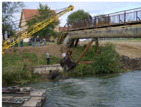
Photo 1. Dredging on upstream Bega channel
