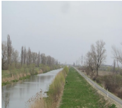
Figure 9. Bega bicycle track
