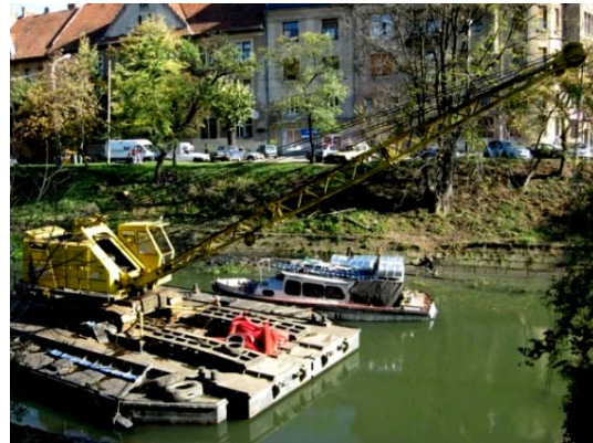
Figure 8. Dredging the Bega Channel
