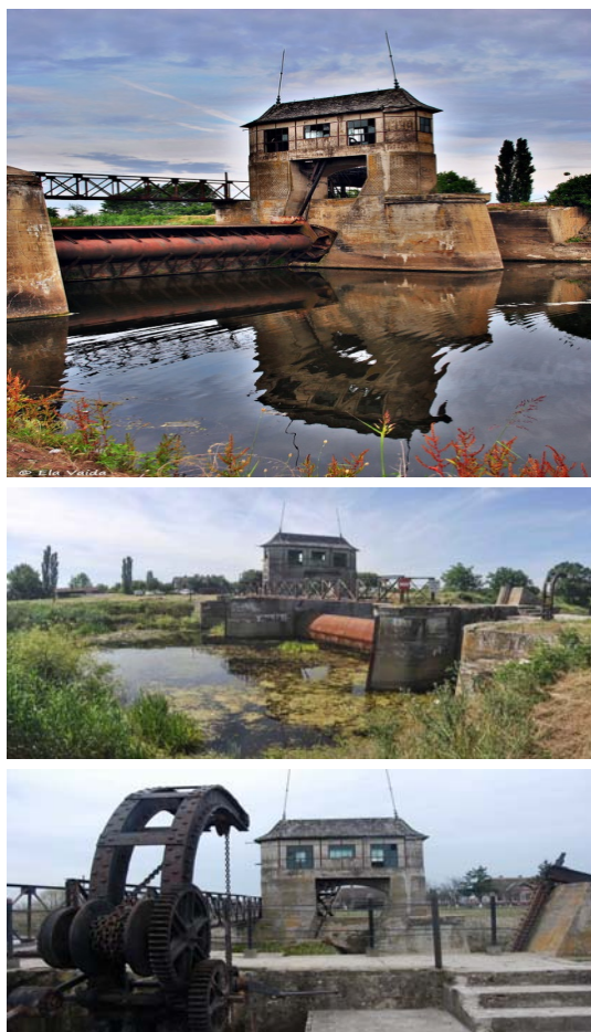
Figure 13. Sanmihaiu Roman hydrotechnical node
