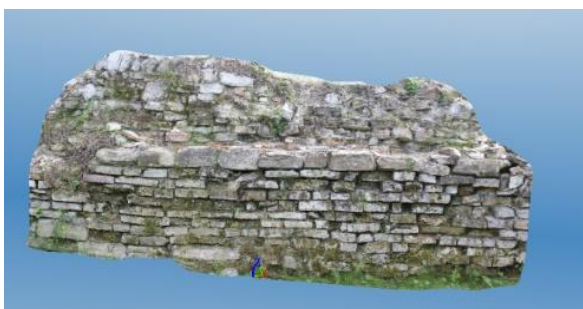
Figure 6. A wall 3D model produced using 123D Catch software [9]
