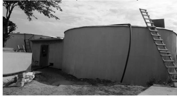
Figure 4. Rehabilitated tanks of 300 cubic meters capacity
