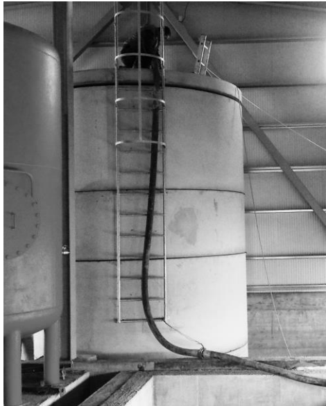
Figure 3. Sequentially decanter for waste water washing
