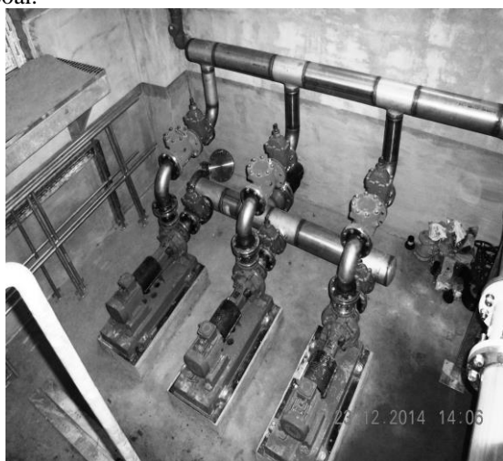
Figure 1. Proposed Treatment Plant - influent pumps / wash filters
