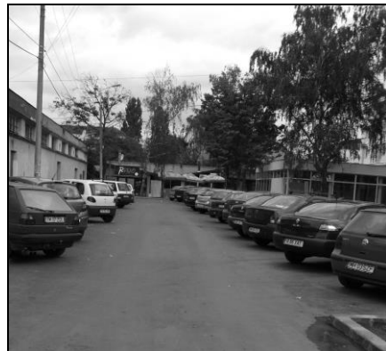
Figure 4. Parking fully waterproofed, Vaida Street, Timisoara
