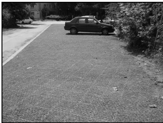
Figure 8. Parking in plastic gratings Șagului Way
