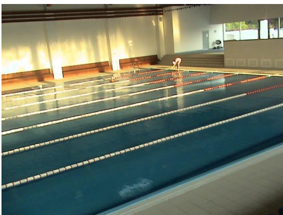
Figure 3 - Water quality and construction of swimming pool T 3
