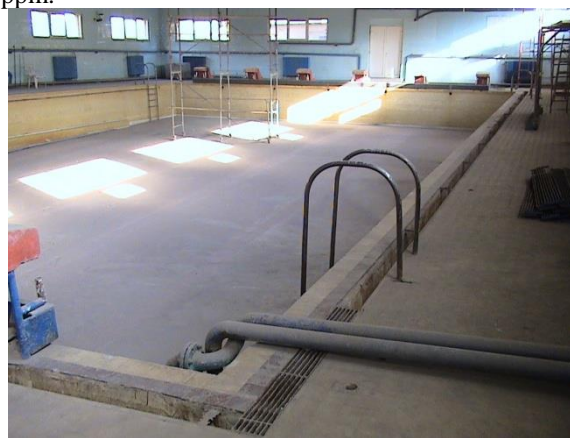
Figure 1 - Construction and installation of swimming pool rehabilitated T 1
