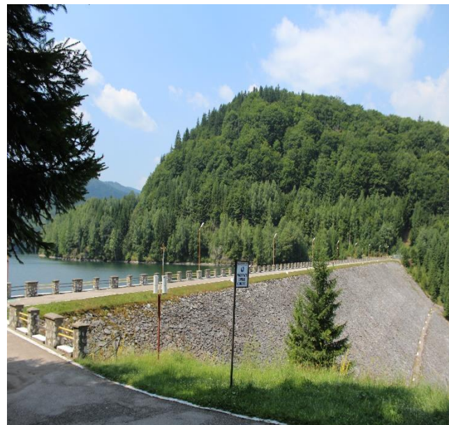
Photo 2. Downstream view - "Valea de Pești" Dam
