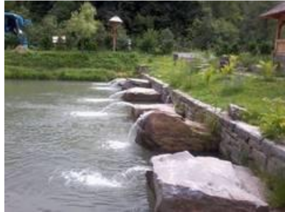
Figure 2. The intake basin
