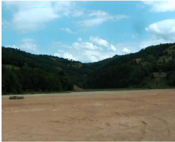
Figure 2. General view of Săliștei Valley pond
