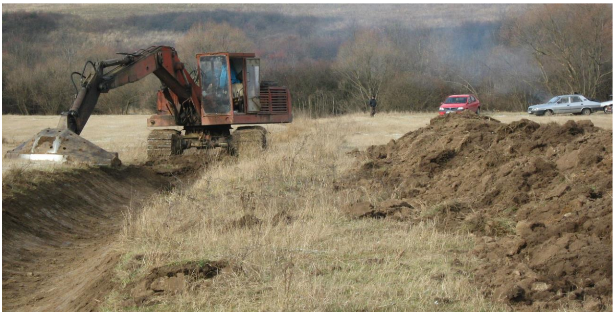
Figure 3. The execution of a channel for the excess water uptake
