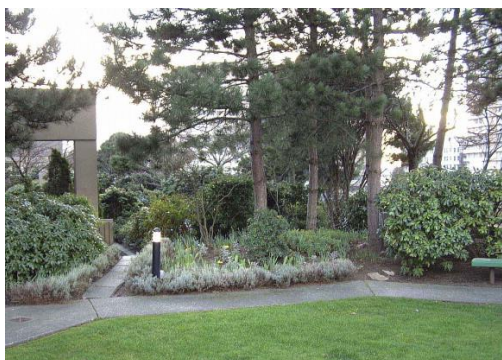
Fig. 17 An intensive green roof on the Coast Plaza Hotel in Vancouver, British Columbia (Photo by Brad Rowe).
