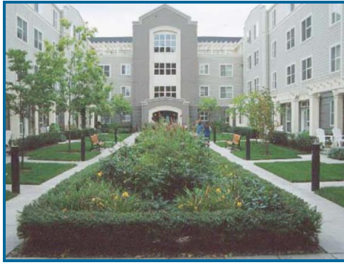
Fig.5: Bioretention area in center of apartment building courtyard, Portland, Oregon [Hinman]
