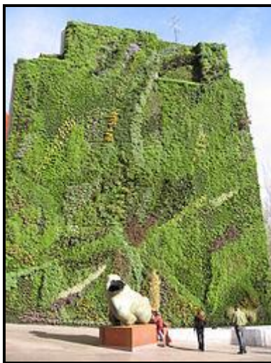
Fig. 16 A wall of living plants designed by Patrick Blanc at Caixa Forum near Atocha station, Madrid.
