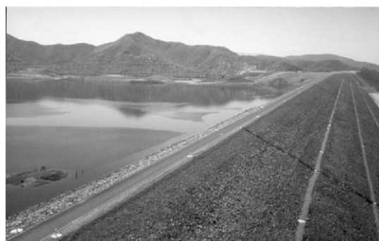
Figure 5. Prisms mounted in the body of the dam
