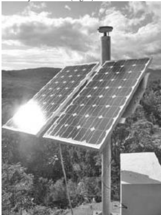
Figure 8. The location of GPS stations and fuel system
