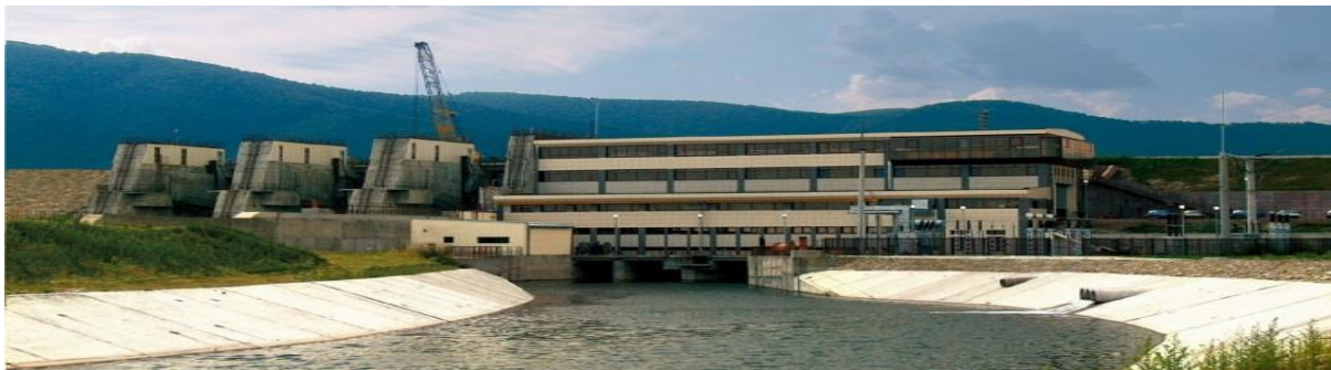
Figure 2. Dam and HEP Subcetate
