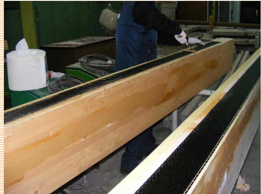
**CONSOLIDATION WITH FRP OF GLUED-LAMINATED TIMBER BEAMS**
