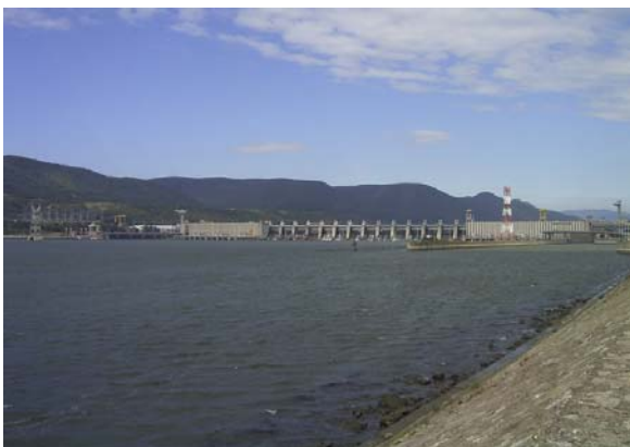
Iron Gate I Hydroelectric Power Station
