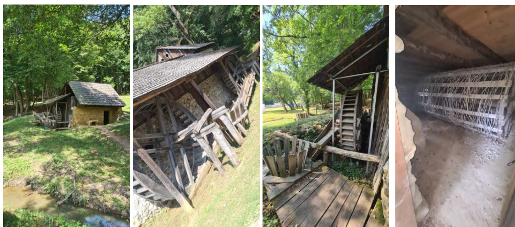
Figure 6. Darsta with two fulling cylinders and two whirlpools from Lucarcesti
