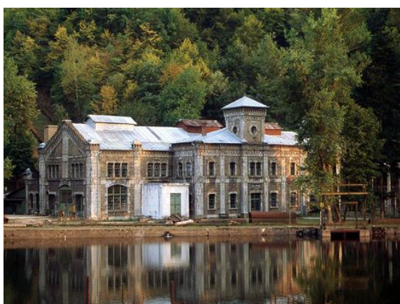
Figure 2. Grebla HPS main building, prior the rehabilitation
