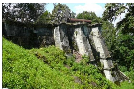
Figure 6. View of the Ranchina surge tank
