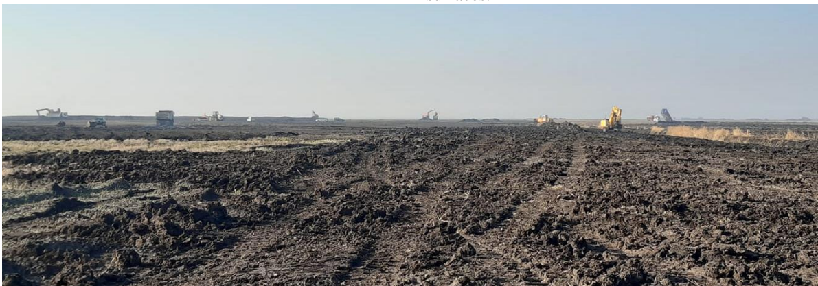
Figure 9. Image during the execution of earthworks [Foto. Ilca M.V]
