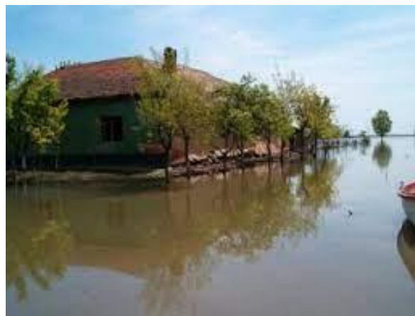
Figure 1b. Flooded street in Foeni commune, Timiș County
