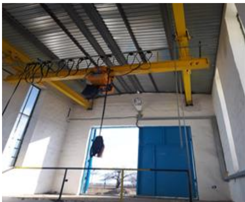
Figure 9. Interior view SPP10 after the rehabilitation of the infrastructure (Photo Cioclov)
