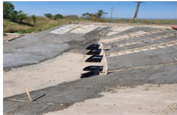
Figure 7. Suction basin view after rehabilitation (Photo Cioclov)
