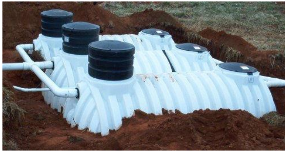
Fig. 5 Below ground tank (Image courtesy Rainwater Management Solutions)
