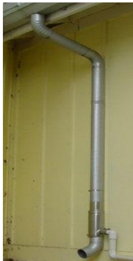
Fig. 2 Downspout (Hans Otto-Wack)
